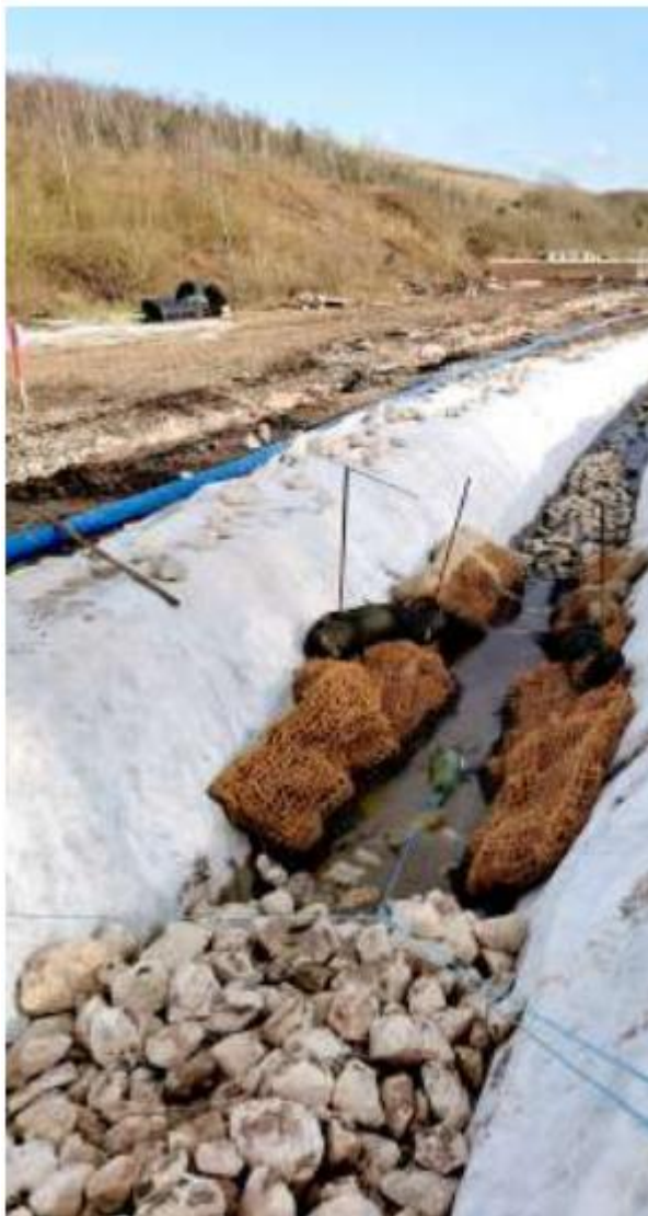
Trench arrangement with turbulence medium, gel flocculant block and silt matting
